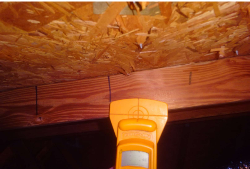
Nail location verified
