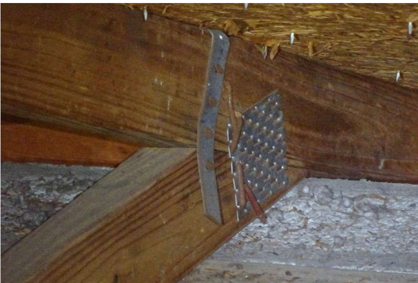
Single wrap with at least 2 nails in the embedded side and at least 1 nail in the wrapped side
